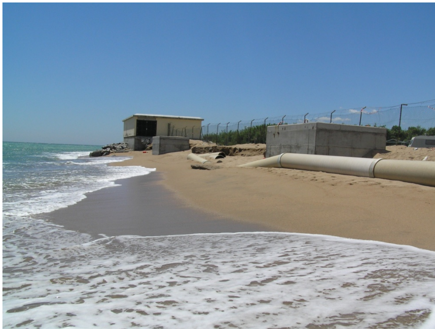
Figure 56. Auxiliary installations of a desalination plant in Blanes (Catalonia, Spain) exposed to wave action due to coastal erosion.
